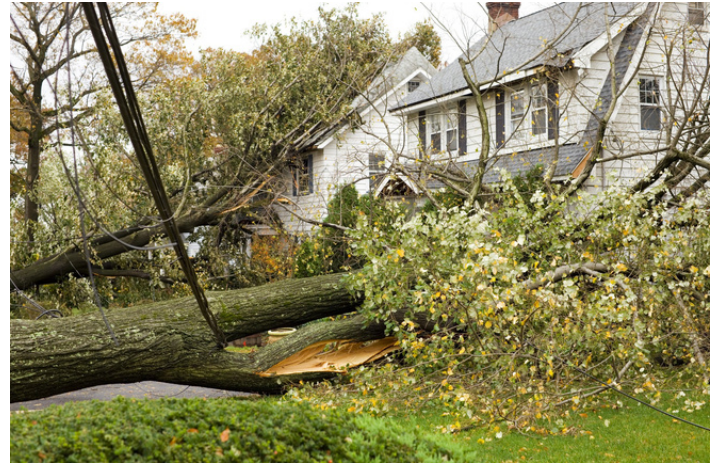
Emergency Disaster Relief
